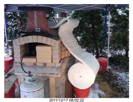
I removed the tent for safety when working with the Insulfrax blankets I purchased from Forno Bravo.
