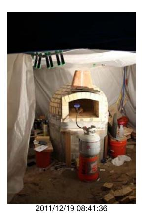
I cured the oven with propane burner from Cajun Cooker. This worked well.
