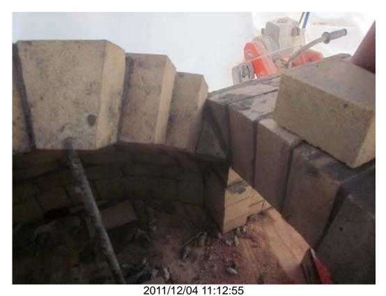
I cut dome "voussoirs" tapered in both dimensions. Forno Bravo forum was huge help in predicting angles. I did trial and error at first with OK results.
