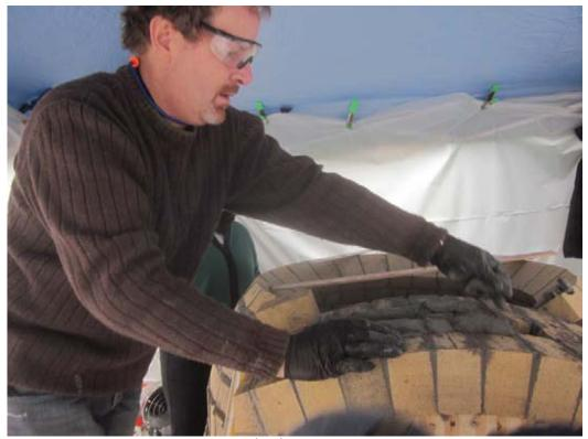
2011/12/03 14:52:19 Used the smallest flue Superior Clay made (4.5" x 8.5"). Cut bottom pieces to form taper to single upper flue.
