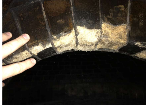
Arch bricks disintegrating
