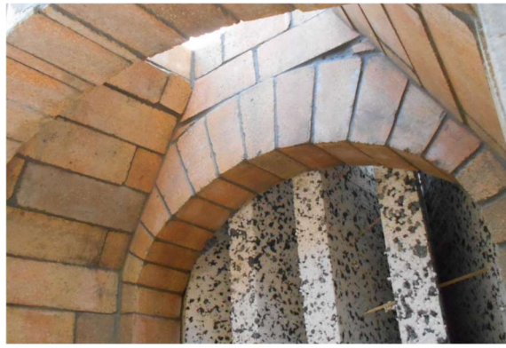
Arch bricks when built
