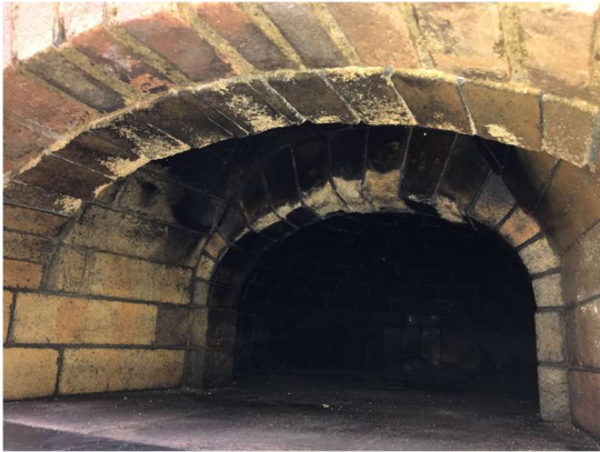
Arch bricks disintegrating
